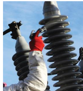
Spraying the HVIC coating on site
