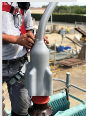
Installing the E/COVER on an insulator
