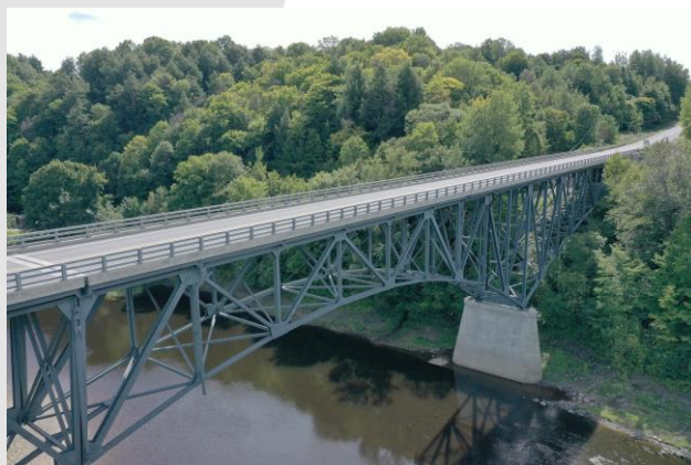
Corrosion protection for major structures
