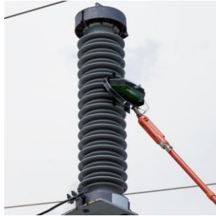
Electrical substation insulator tester
