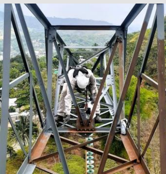
Application of GALVAGRID® coating
