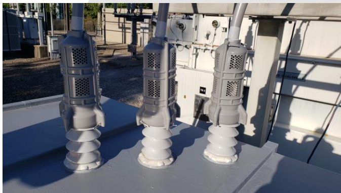
E/COVERBIRD Silicone covers for thermography and bird protection
