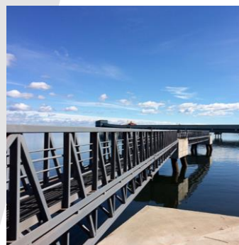
Protection of steel structures up to C5H
