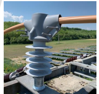
E/COVER Removable insulating covers
