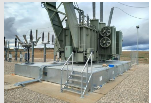
ERT-MODULO 5 tank with access stairs
