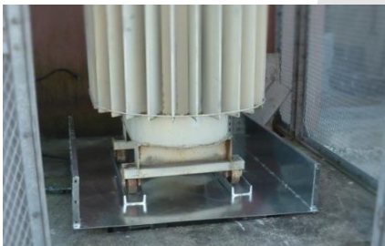
BDRG2 drip tray with open side panel and transformer roll-out
