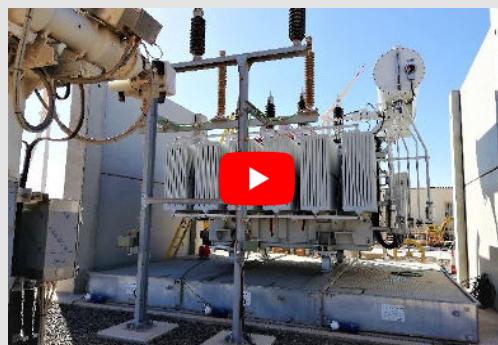
TRT®-LHD-MODULO 3 extinguishing retention tank with SP® filtration system
