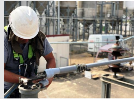
3 Press firmly on the tape to remove air pockets.
