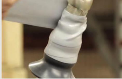
2 Apply a second wrap for 35 kV insulation.
